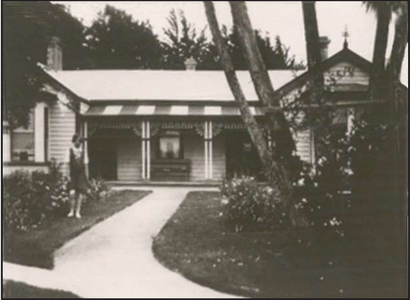
The new timber house at Thornbury
