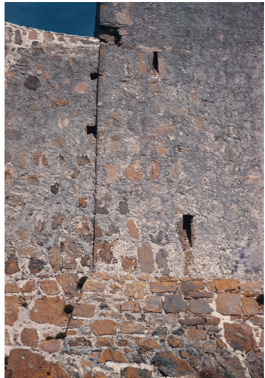
ILLUS 8 Straight butt joint between castle and curtain wall suggesting the curtain to be the secondary structure (Macneil Collection 1960s, S153, © Crown Copyright: HES)
