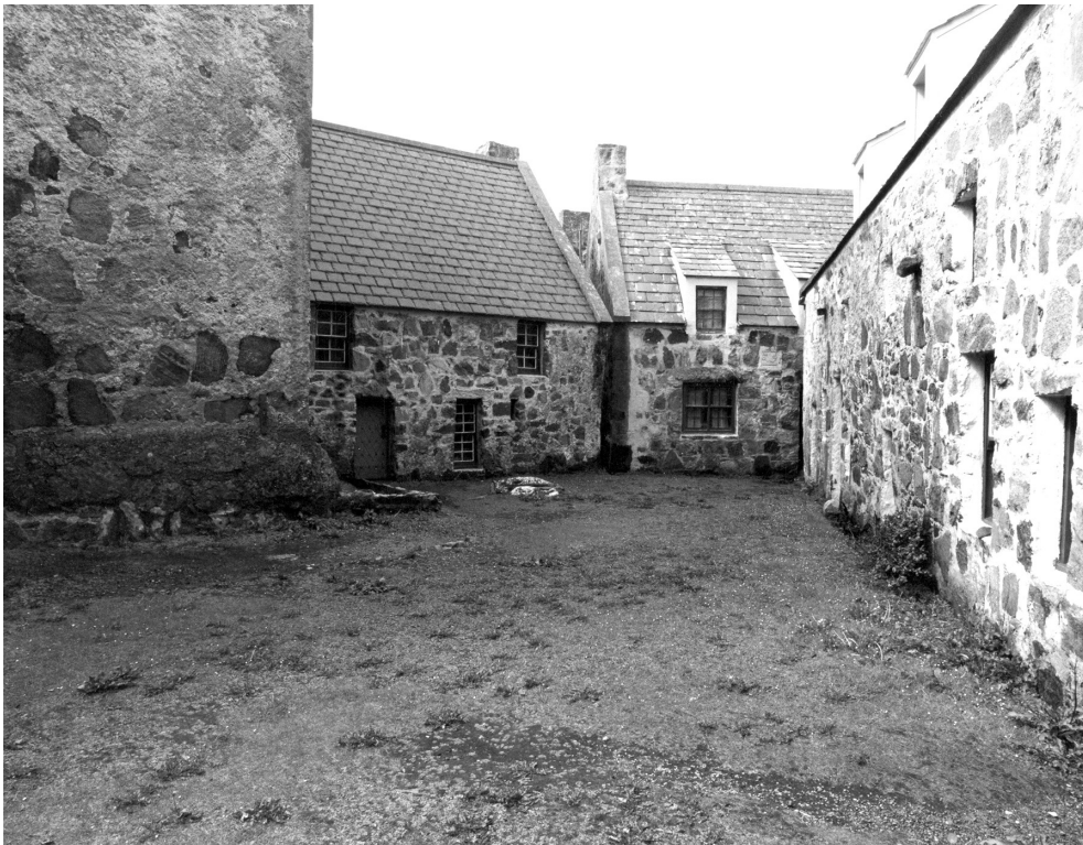
ILLUS 12 The courtyard looking towards the restored kitchen and the Tanist house (© Crown Copyright: HES)
