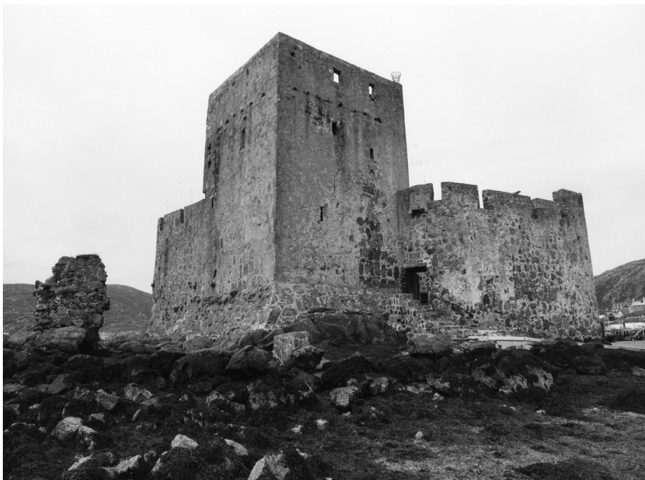
ILLUS 4 The castle from the south-east (© Crown Copyright: HES)
