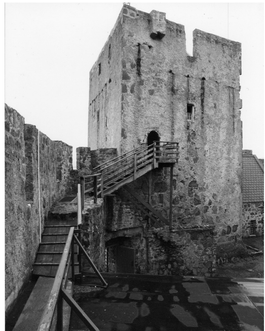
ILLUS 7 The tower and curtain wall from the north-east showing the castle entrance and current arrangement of forestair and gantry that gives access to the first floor (© Crown Copyright: HES)
